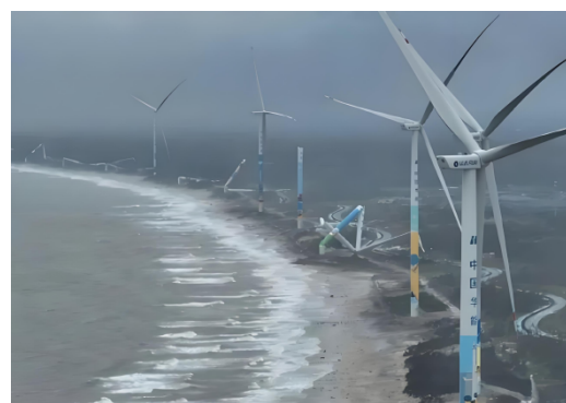
Fig. 1.9 (f) Wind turbine tower losses in Hainan
